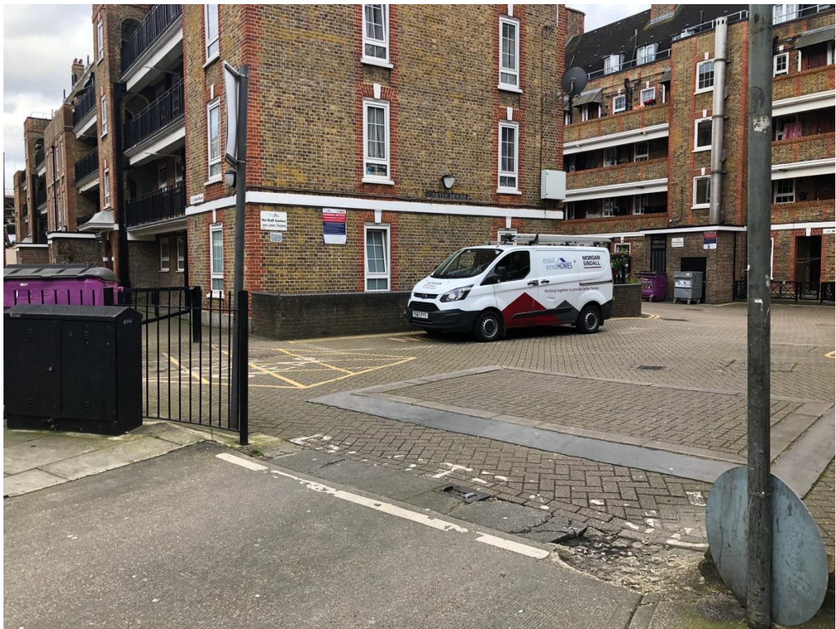
View 1: Looking south at the vehicular access on Brune Street
