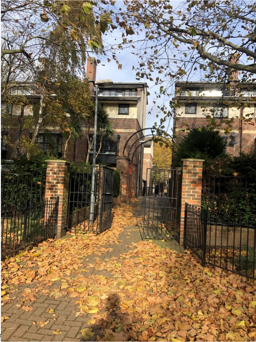
Photo 1 – Looking north at the approved gates at the southern entrance of the passage:
